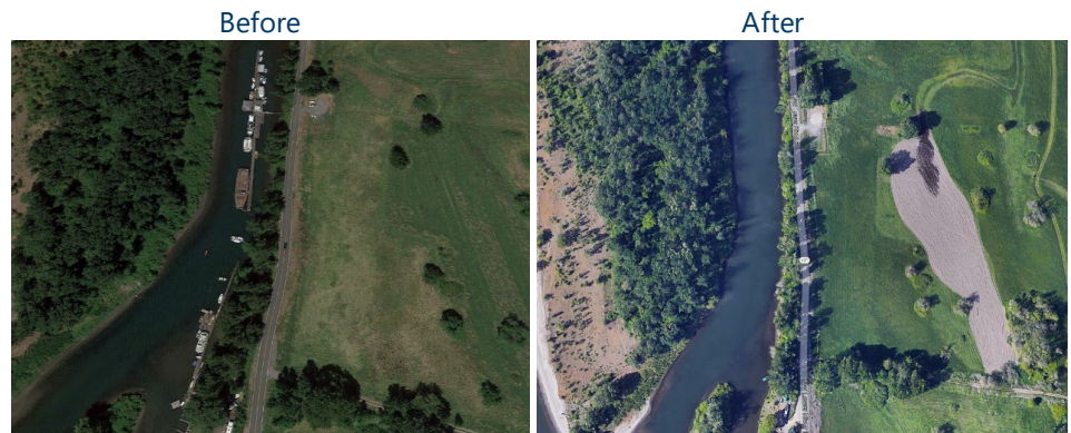
Finished Project: Fisherman’s Slough, Columbia River
