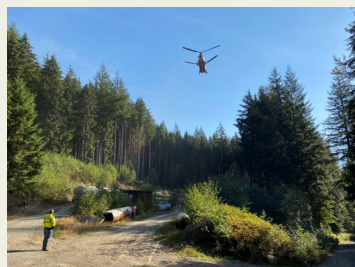
Helicopter bridge installation
