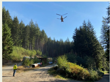
Helicopter bridge installation
