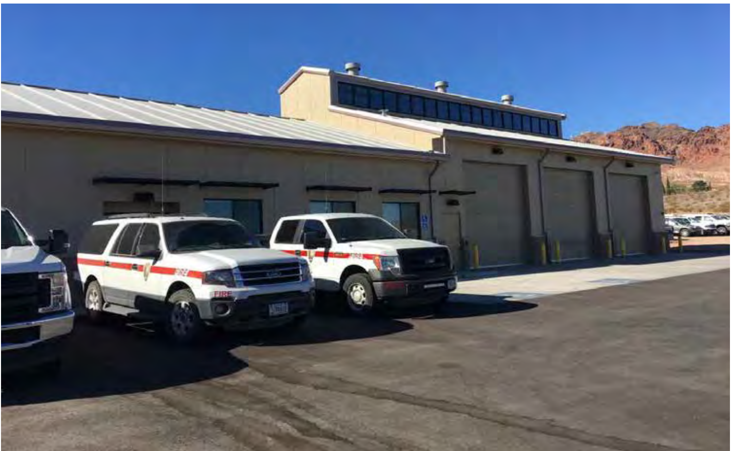
A new fire facility at Lake Mead National Recreation Area replaces makeshift facilities used in the past.
