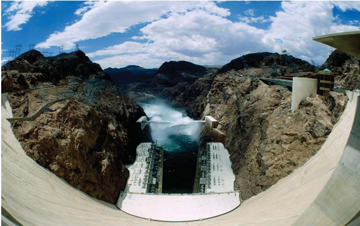
View from Hoover Dam crest during test of jet flow gates
