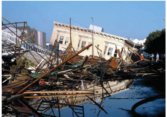
Loma Prieta earthquake, Beach and Divisadero Streets, Marina District, San Francisco, California, October 1989
