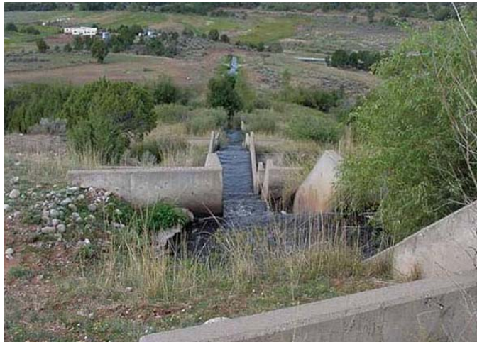
Drop Structure – Pine River Irrigation Project
