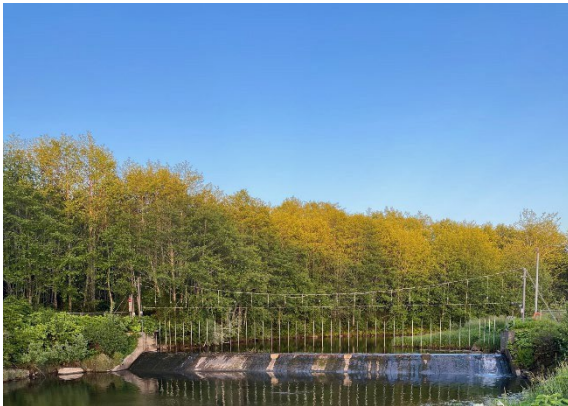
The Makah NFH fish weir before repairs.
