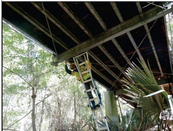
Hands-On Inspection of NSTM of the Iron Bridge at Tensas River National Wildlife Refuge, Louisiana
