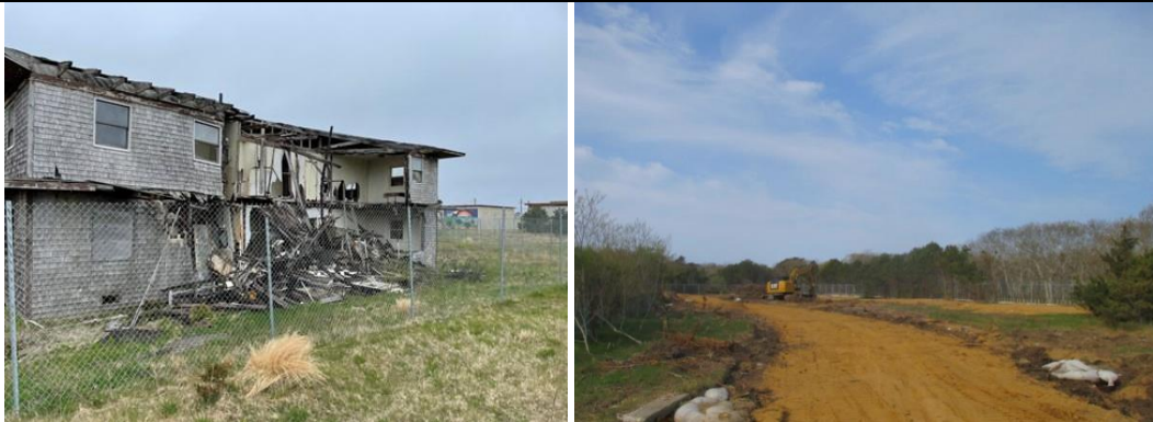
Left: Dilapidated Highlands Center building
