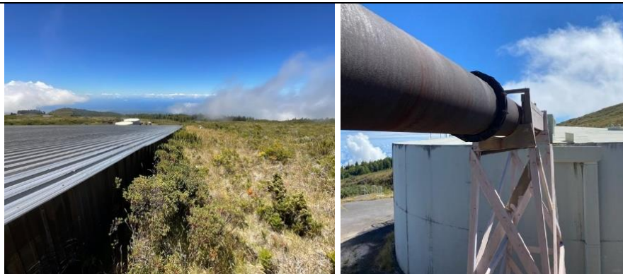
Left: Rain Catchment Structure Right: Water Piping and Storage
