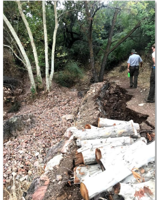
Before Rehabilitation: Flood damage after the Woodbury Fire in 2019 caused a trail to degrade. (Photo by NPS)
