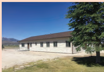
The Weaver Mountain fire facility in the Bureau of Land Management's Phoenix District was a multiyear, multiphased project completed in 2018. It will benefit fire response operations as well as firefighter recruitment and retention efforts. Photo by the Bureau of Land Management.
