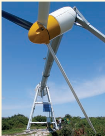
The 80-foot Appledore Island wind turbine can be lowered at the flick of a switch.
