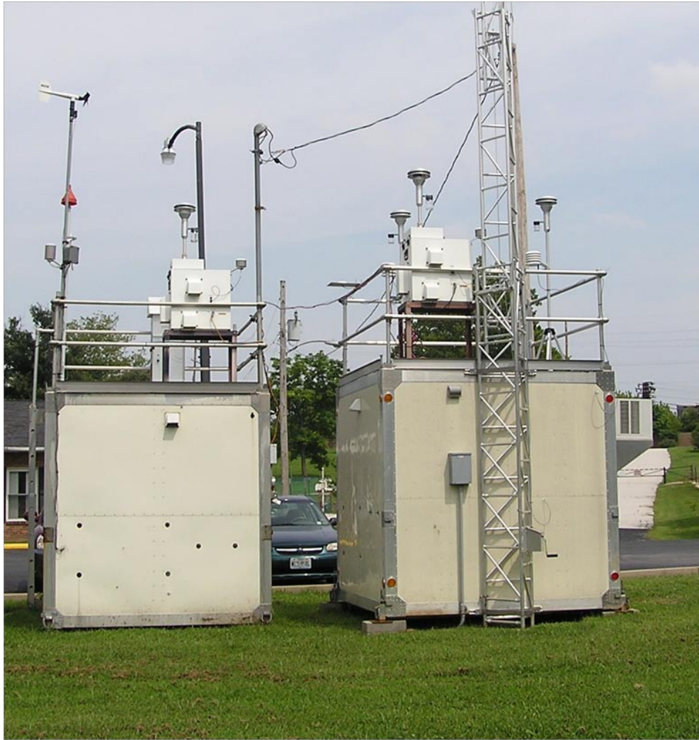
Figure 4. Photograph showing air conditioned monitoring sheds used to house an Xact FLM in Herculaneum, MO.
