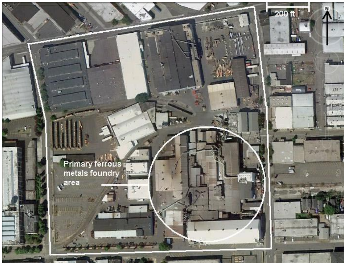
Figure 5. Ferrous Metals Foundry Aerial Map
