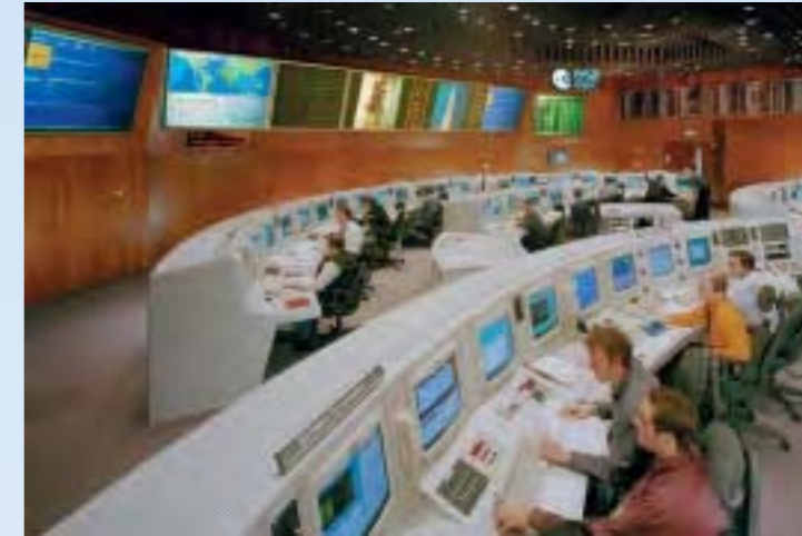
The main control room in ESOC.
