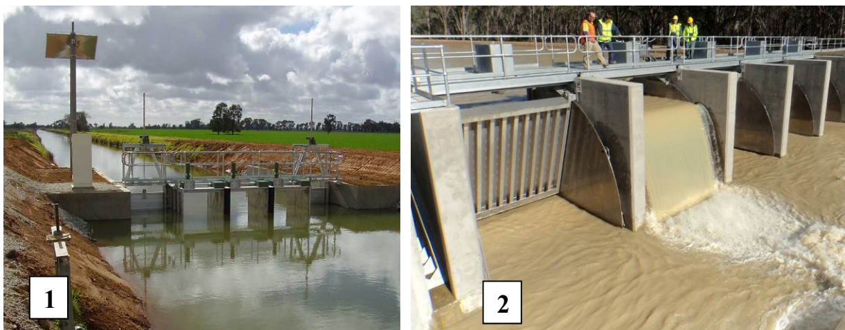
Figure 11: Undershot (left) and overshot (right) regulators. Both impact upstream migration, but undershot regulators have been demonstrated to impact downstream migrating fish, resulting from impacts, barotrauma and shear stresses. (Photo credit: AWMA, Pty. Ltd, Australia.)
