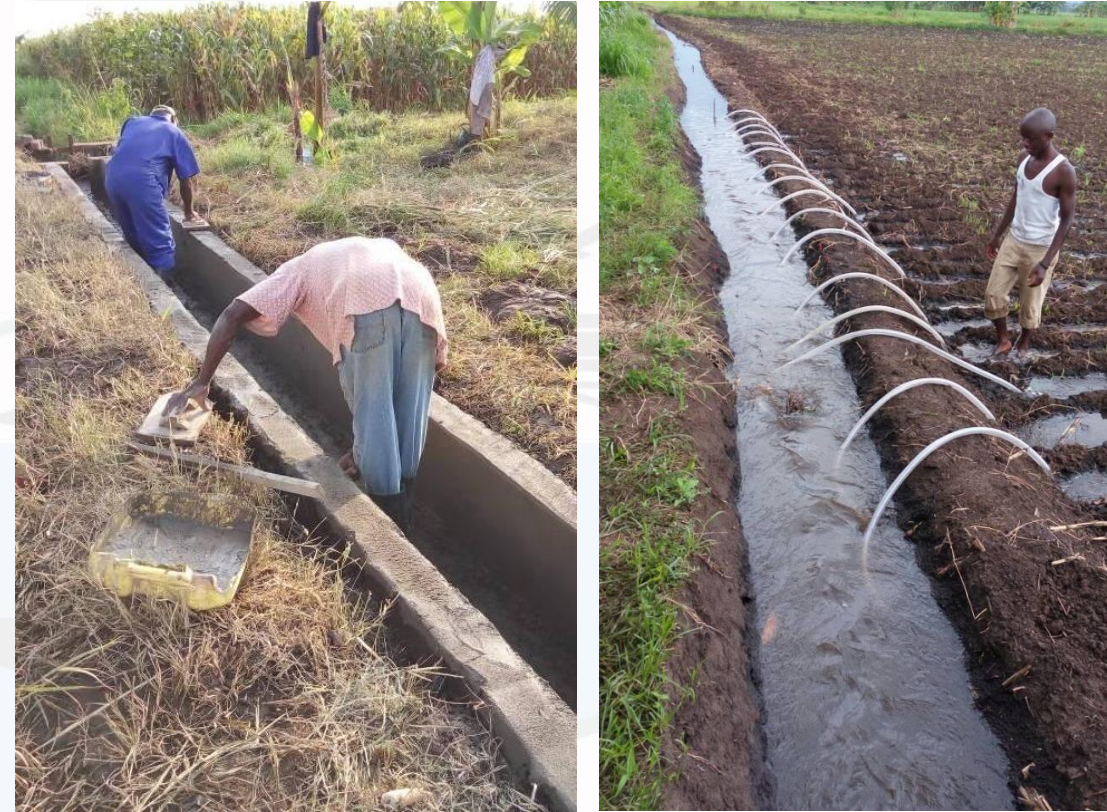
Fig.8: Improved Tertiary and Field Canals.
