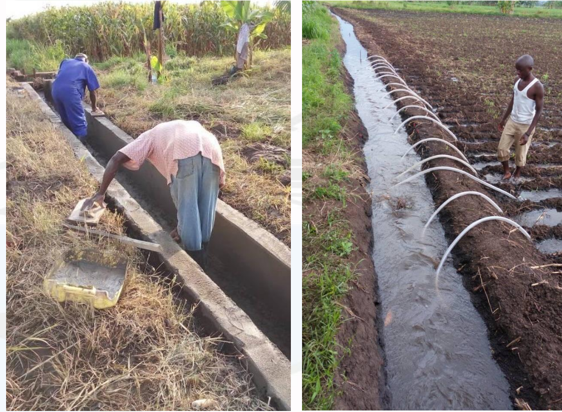
Fig.5: Improved Tertiary and Field Canals.
