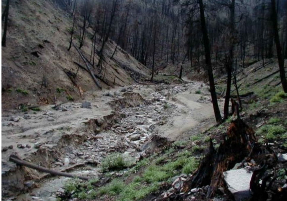
Figure 3-5: Post-wildfire channel for debris flow in John Day, Oregon.
