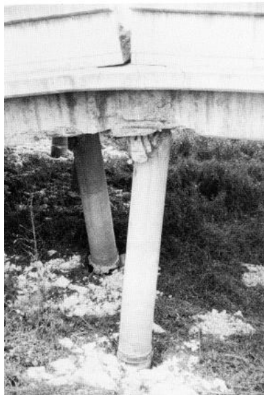
Figure 10-3 Piles Punched-Through the Deck Slab in the Collapsed Struve Slough Bridge (EERI, 1990)
