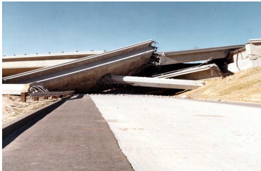
Figure 1-4 Collapse of the I-5, SR-14 Overpass in the 1971 San Fernando Earthquake (USGS)
