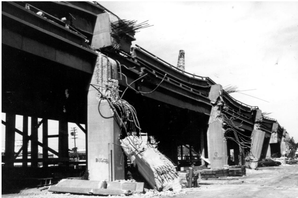
Figure 1-3 Collapse of the Cypress Viaduct in the 1989 Loma Prieta Earthquake (USGS)
