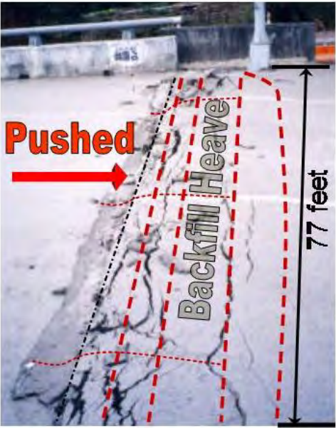
Figure 12-6 Formations of Mobilized Passive Wedges (Kosa et al., 2001)
