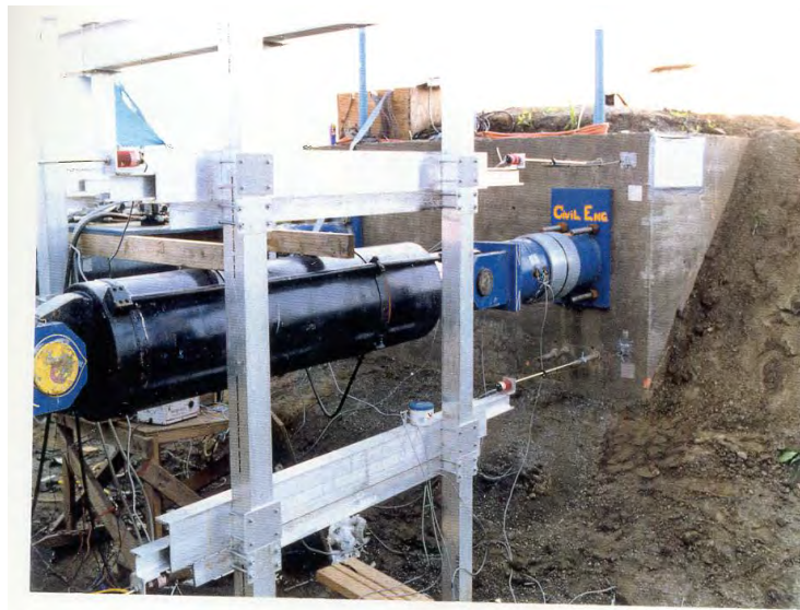
Figure 12-10 UCD Abutment Test Loading Setup
