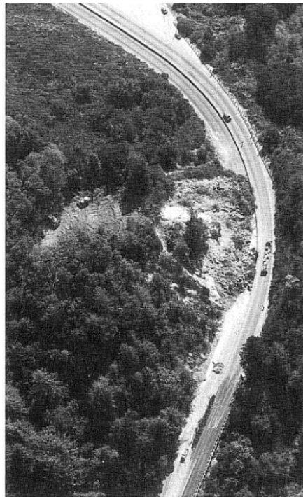
Figure 7-2 Route 17 landslide, Loma Prieta Earthquake (after USGS, 1998a)
