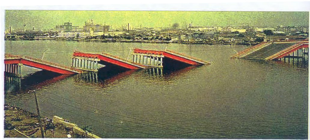
Figure 7-15 Showa Bridge Collapse (Hamada, 1992)
