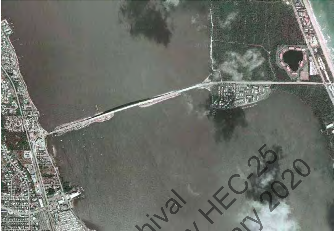
Figure 9.10. Jensen Beach Causeway bridge.
