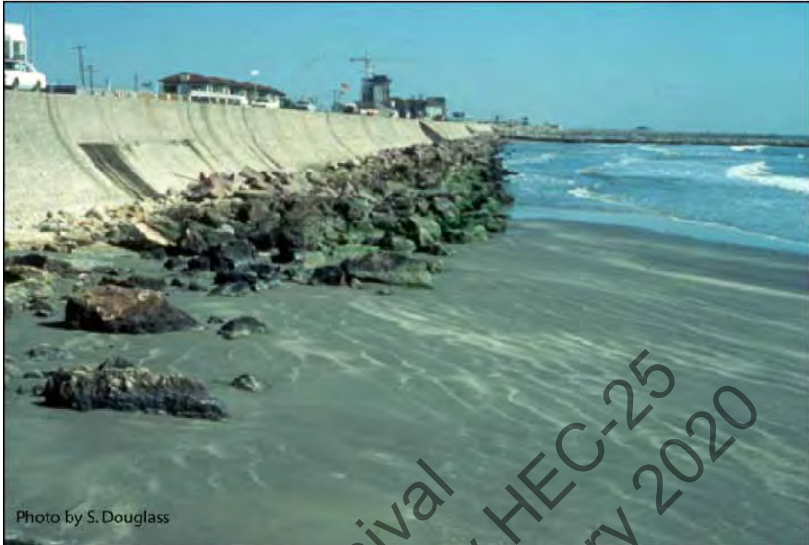
Figure 6.3. Galveston Seawall, Seawall Boulevard (1983)
