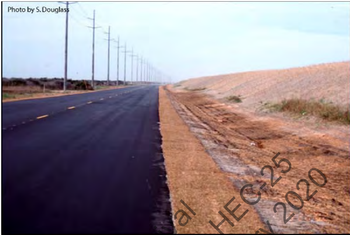
Figure 8.18. Artificial sand dune constructed seaward of a highway to protect the highway (North Carolina Highway 12)
