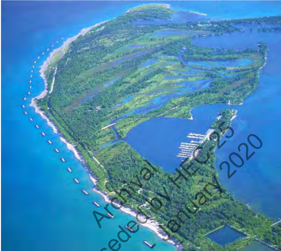
Figure 7.20. Offshore segmented breakwater system at Presque Isle, Pennsylvania
