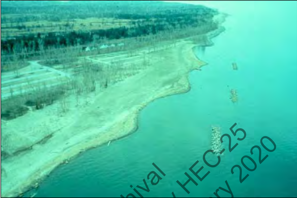
Figure 7.19. Offshore segmented breakwaters with salients in beach nourishment (USACE archive photo, circa 1980).
