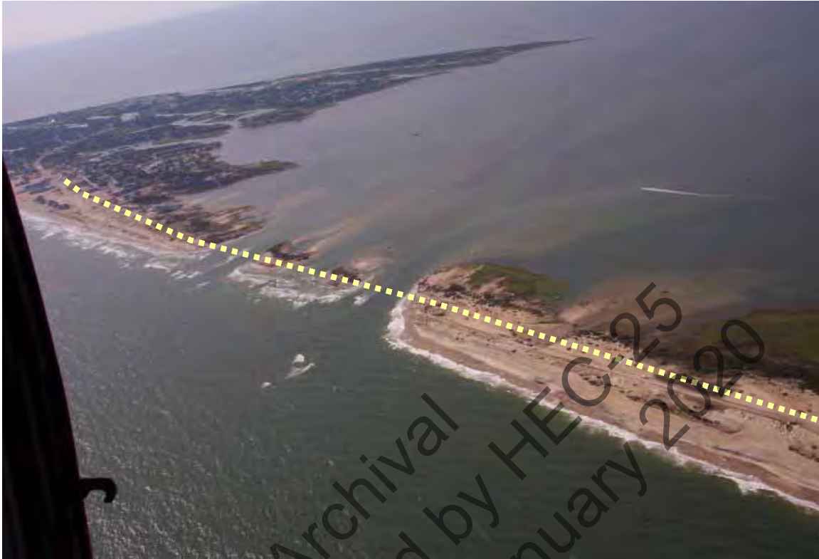
Figure 2.6. Breaches in Outer Bank barrier island caused by Hurricane Isabel in 2002 (NC 12 ROW is dotted line).
