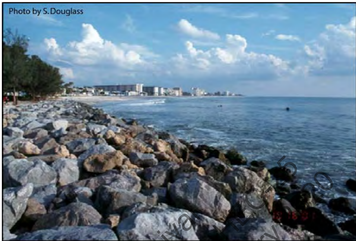
Figure 6.5. Seawall protecting a coastal highway. Venice, Florida (2001)
