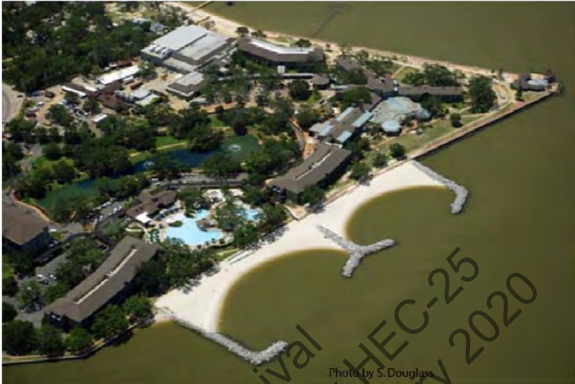
Figure 7.23. Constructed pocket beach stabilized with a T-head groin breakwater system (Point Clear, Alabama).
