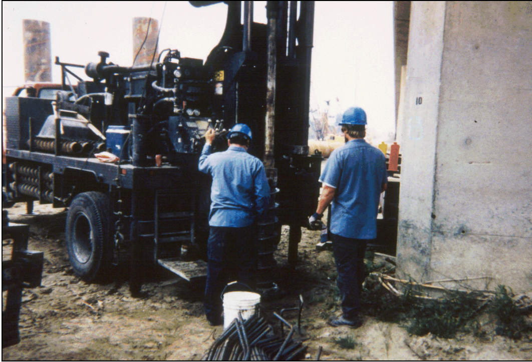
Figure 9.29. CALTRANS drilling with hollow stem auger for installation of float out devices at Salinas River Bridge (Highway 101) near Soledad, CA.
