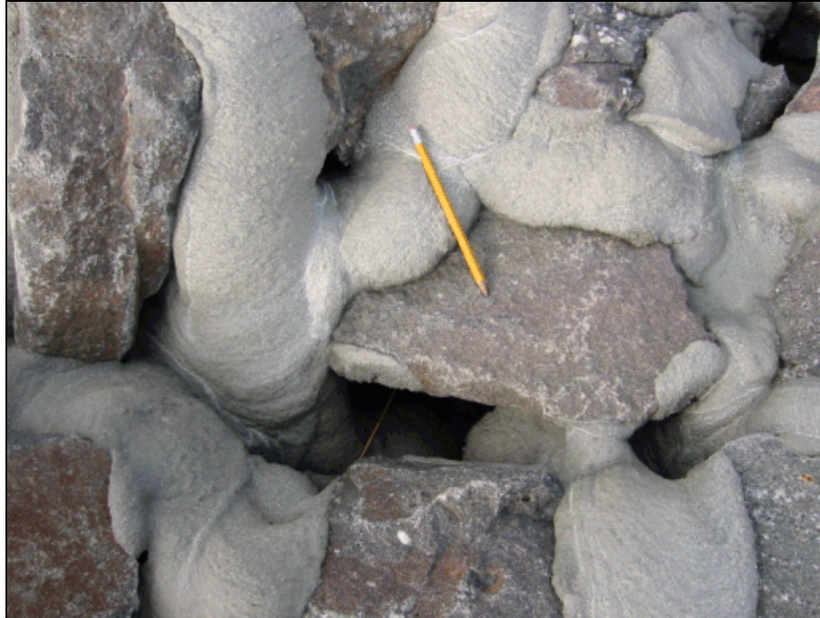
Figure 5.20. Close-up view of partially grouted riprap.
