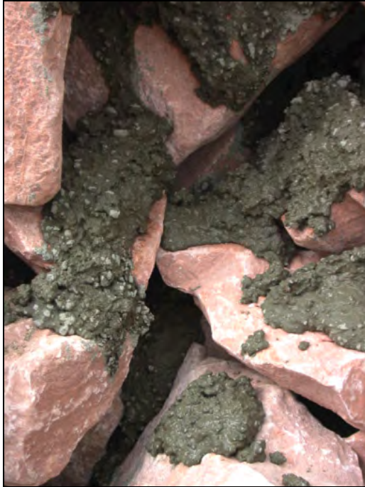
Figure 12.10. Interior of the dry riprap pile (some surface rocks removed).
