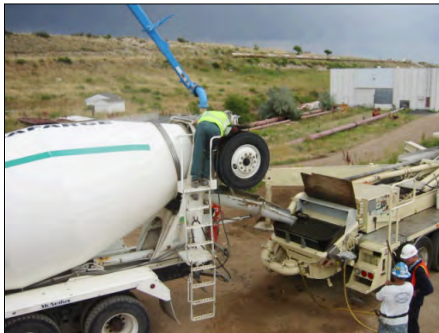
Figure 12.7. Concrete mixer truck and pump truck with boom.
