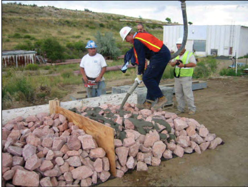
Figure 12.8. Preliminary trial grout application in the dry.
