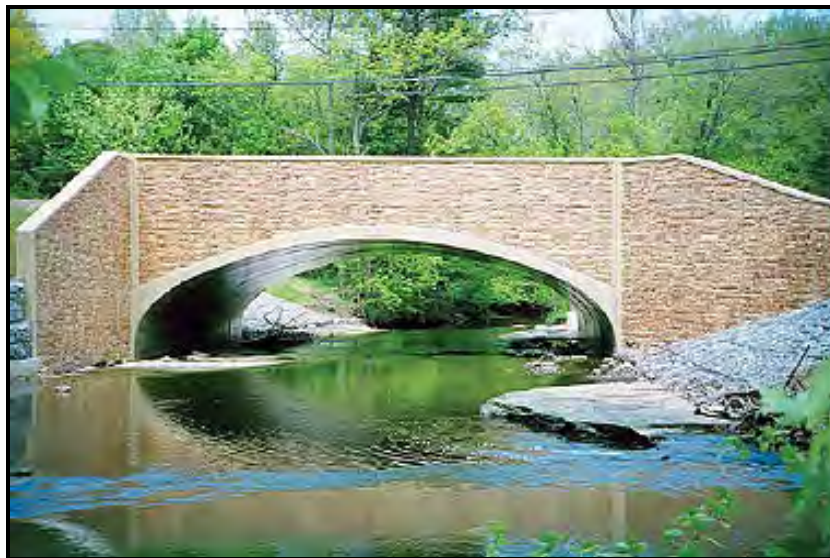
Figure 18.1 Bottomless Culvert on Whitehall Road over Euclid Creek in Cuyahoga County, OH.
