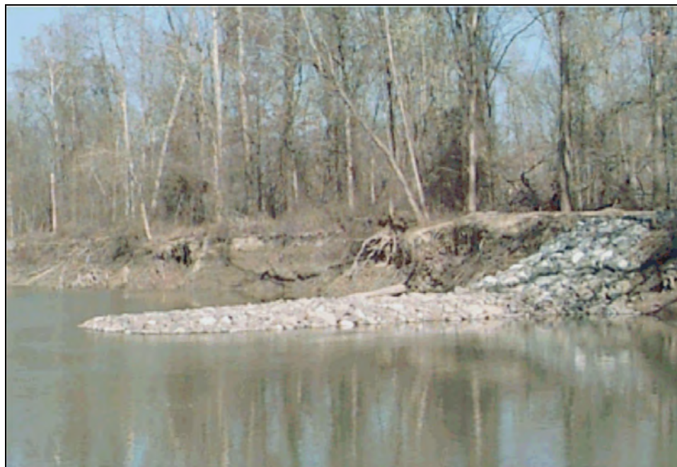
Figure 1.10. Close up bendway weir on Hatchie River (TDOT).
