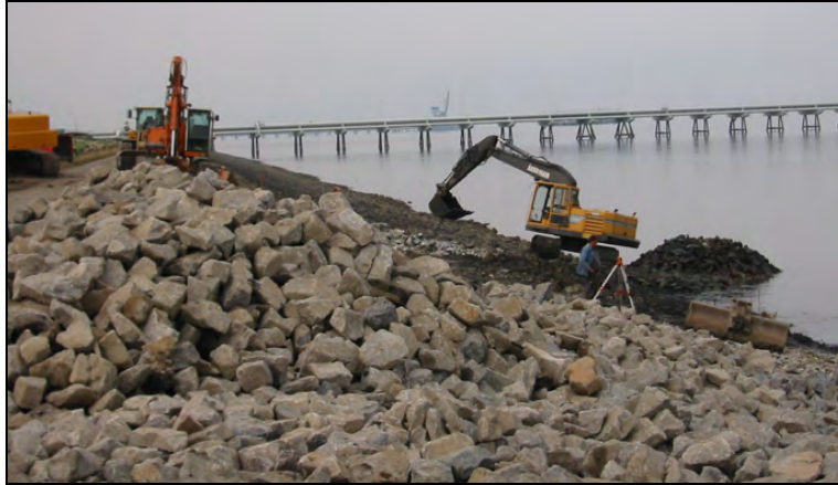
Figure 12.18. Placing riprap with hydraulic excavators.
