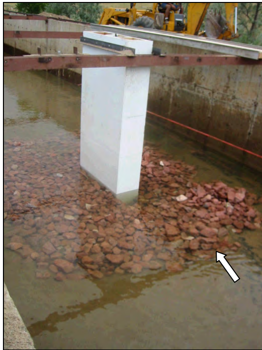
Figure 11.14. Riprap armor over geotextile containers.
