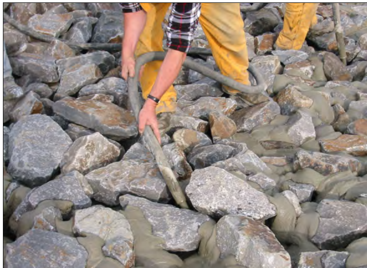
Figure 12.20. Grout placement by hand.
