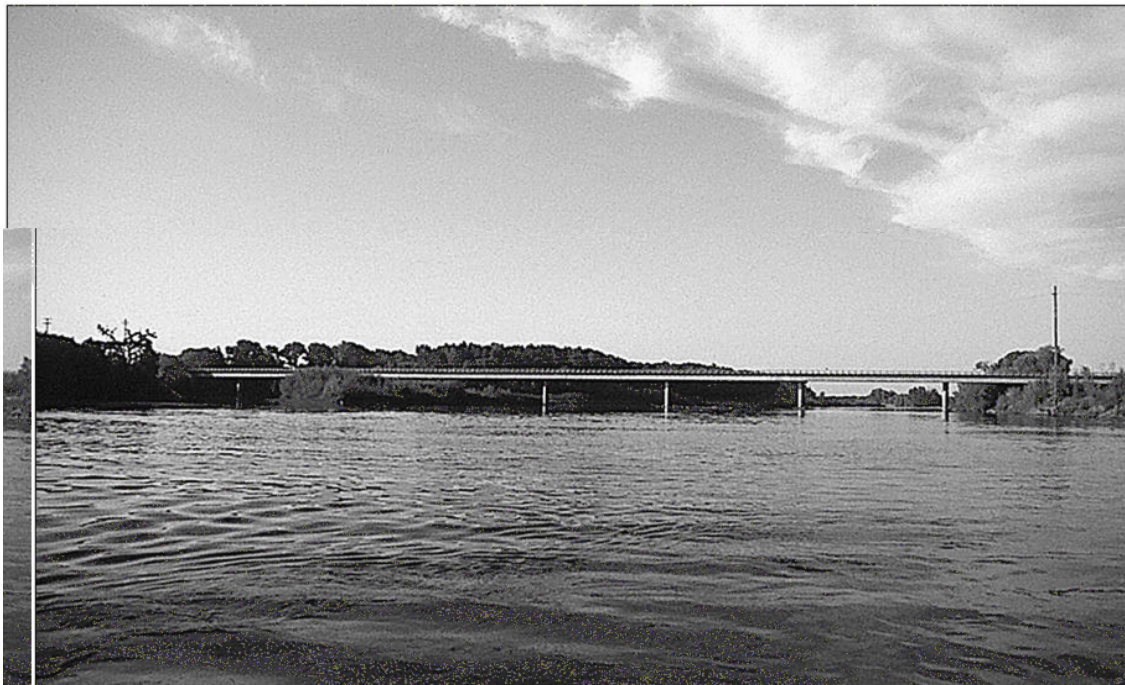
Figure D.2. View of Ordbend bridge looking upstream showing bridge characteristics.
