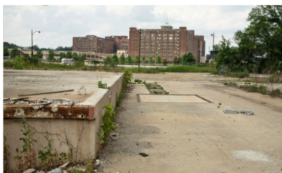
Before Atlanta BeltLine Construction
