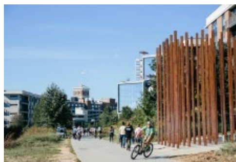
After Atlanta BeltLine Construction
