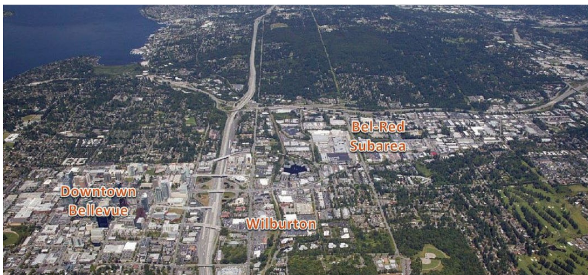
Figure 20. Aerial View of Bel-Red Subarea
