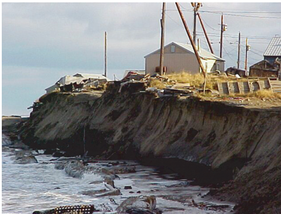
Figure 9: Bluff Erosion and Permafrost Melting in Shishmaref (c. 2002)
