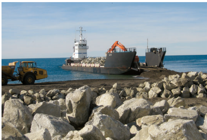
Unloading rocks for Kivalina's seawall
