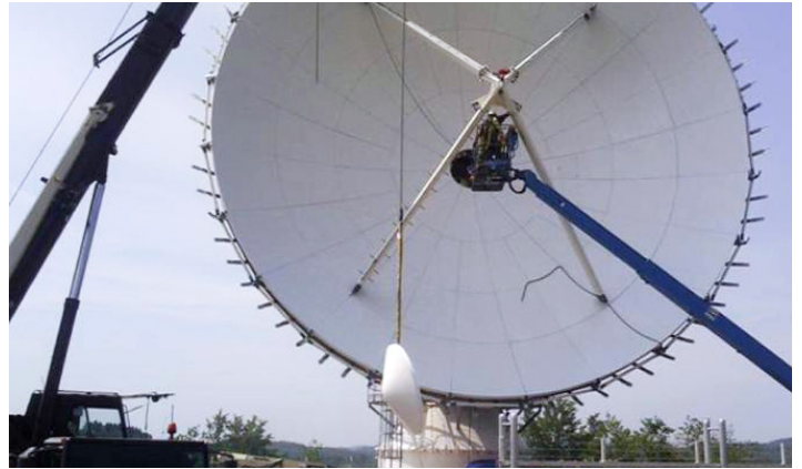
GOES-R RBU Antenna Construction
