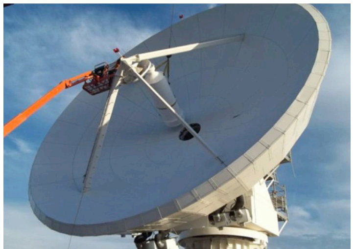
Antenna feed installation at WCDAS. Credit: Harris Corporation
