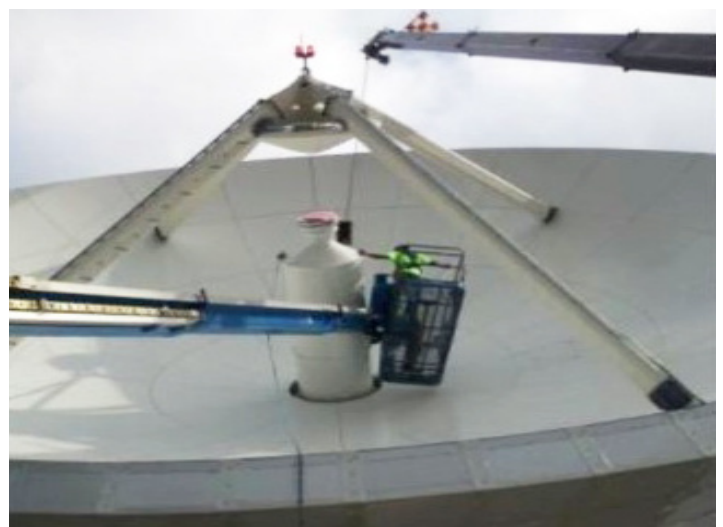
RBU R-2 antenna feed installation. Credit: Harris Corporation
