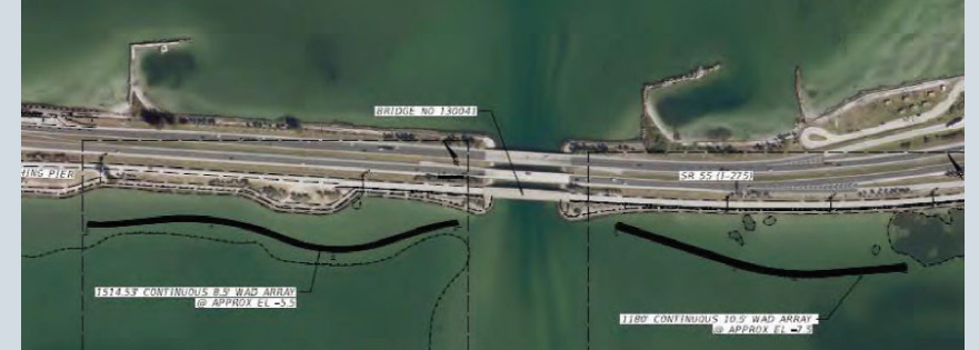
Sunshine Skyway Wave Attenuation Units (WADs) (2023)
