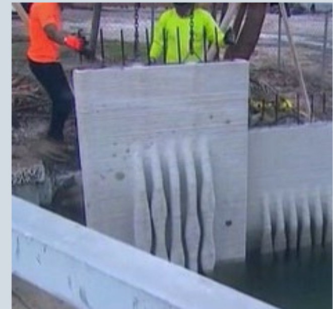
Kind Design Living Seawalls (Miami Beach, 2024)
