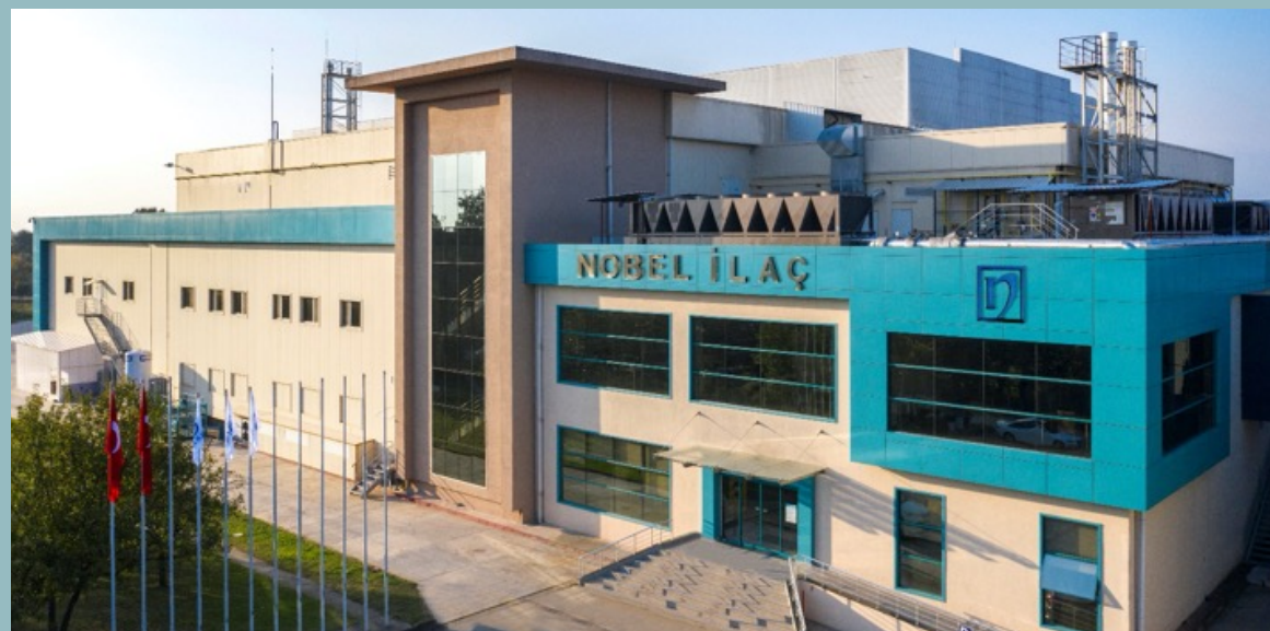
Nobel's facility in Düzce, a small, industrialized city in the Black Sea region between Ankara and Istanbul.
