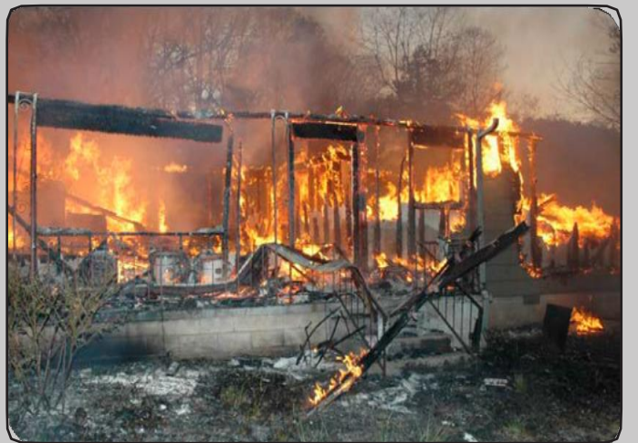
An elderly man died as a result of this fire in south Knox County
