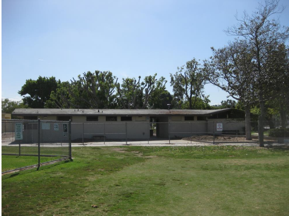
Plate 9. Restroom Facility, north side, view facing south
