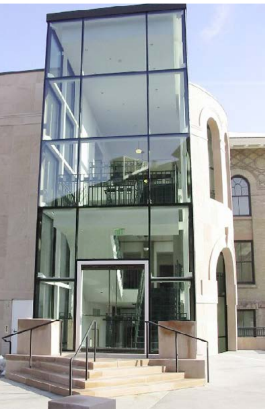
Completed structure connecting Cowles and Widtsoe Buildings
