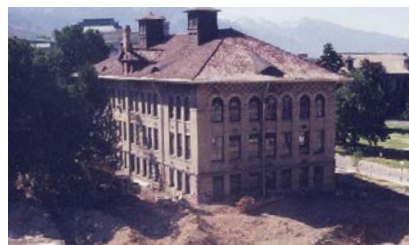
Construction to connect the Widtsoe and Cowles Buildings
