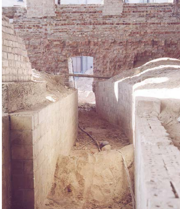
Tunnel showing the foundations of the Cowles Building
