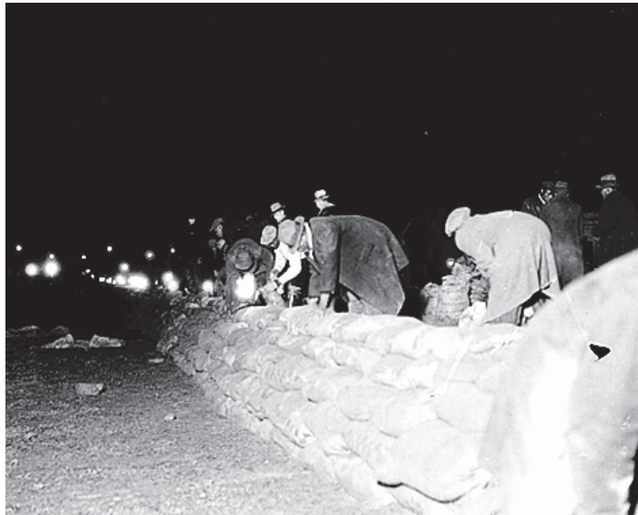
Workmen from the Works Progress Administration (WPA) use sandbags to build an emergency levee against the Great Spring Flood of 1936 in Washington, D.C., the event that led Congress to order the building of a permanent levee along the National Mall. PHOTO, DEPARTMENT OF THE INTERIOR
