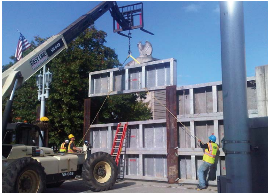
An artist’s sketch shows an early version of the 17th-Street flood wall (left). The photo above shows an example of how a “post-and-panel” flood wall would be erected. The Washington wall will have nine posts and 27 panels, all of them stored off-site. When a major flood event threatens the city, they would be trucked to 17th Street and craned into place. DRAWING AND PHOTO, COURTESY OF THE U.S. ARMY CORPS OF ENGINEERS
