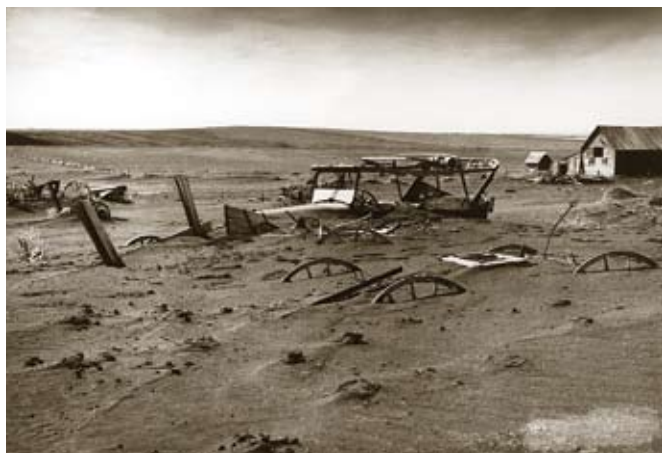
Machinery buried by blowing soil—1936.
