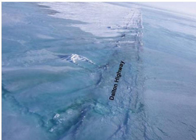
Image courtesy: Department of Transportation and Public Facilities in Alaska. Photo was taken on April 08, 2015 around the inundated Dalton Highway near Sag River.
