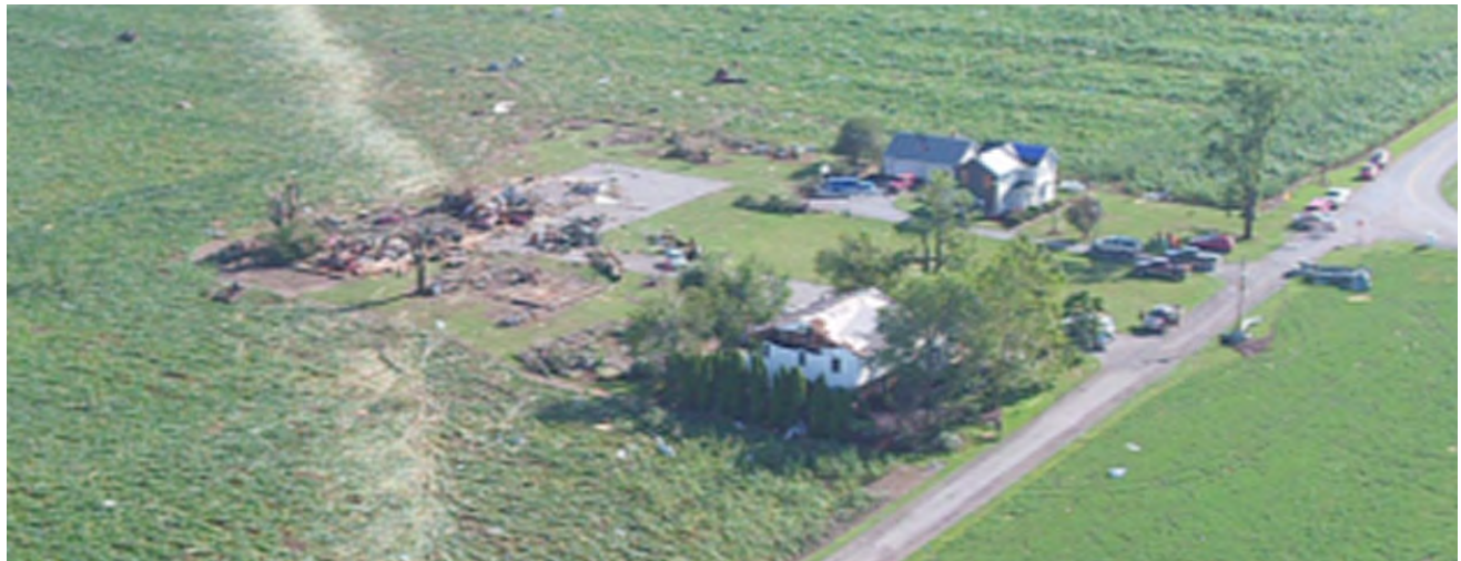
Tornado damage near Roberts/Doty Roads-Woodburn, IN (Scott Jordan Drone Footage/NWS Storm Survey).
