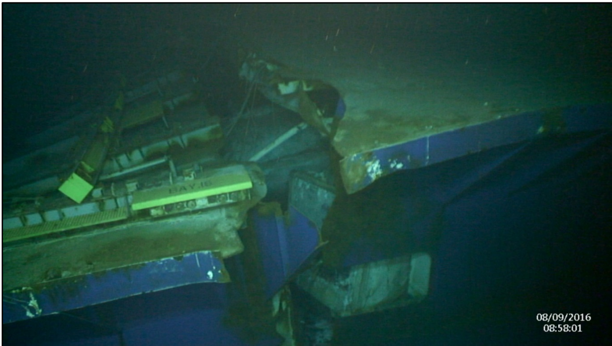
Figure 30. Hull fracture in starboard sideshell and across main deck at container bay 16, forward of frame 200. (Image from mission 3)
