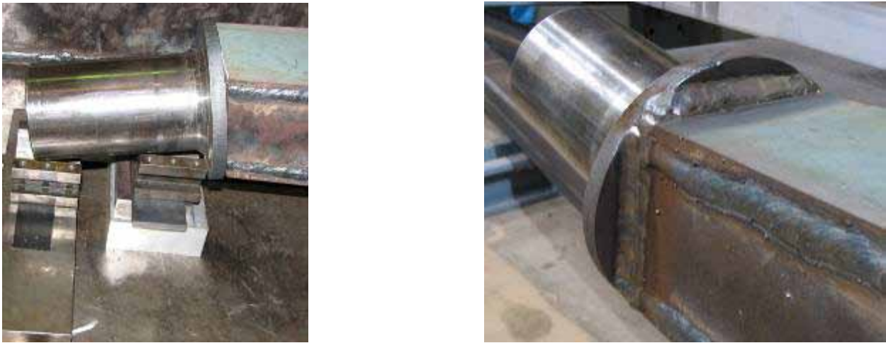
Figure 4.6: Left: End Plate and Axle Shaft are jugged into place for final attachment to the Outboard Beam of the new outriggers. Right: All seams are welded, multiple weld passes maybe necessary. Outboard Beam is complete.
