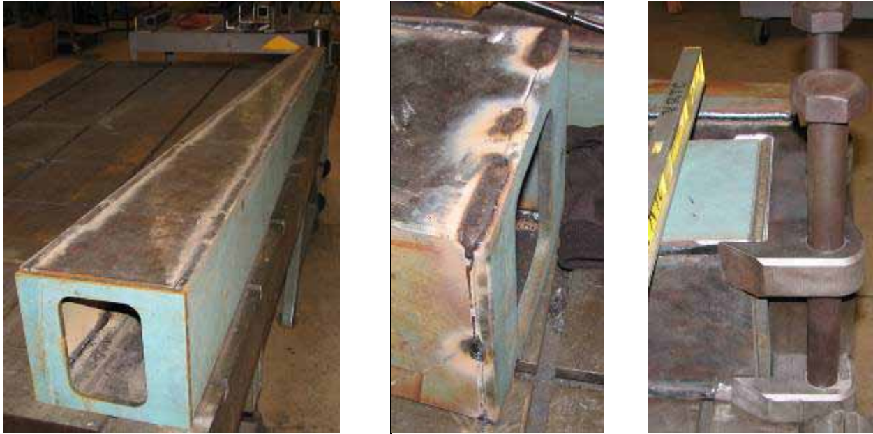
Figure 4.3: Left: Base Plate is added to the end. Middle: Base plate is welded to the Outboard Beam in the locations that the Hinge Brackets will overlap. Right: Hinge Brackets are being jugged up to weld. The bolts shown in the photo were removed and a aluminum jig was inserted into the holes to assure alignment, see Figure 4.4 (Middle).
