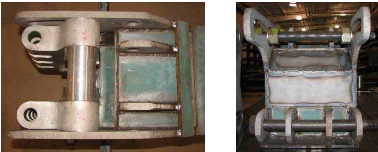
Figure 4.20: Left: 8 th and 9 th steps have been completed and jiggling has been removed. Right: 12 th step has been completed; cover plates were welded in place. Note: Jigs holding the Lower Adjustment Brackets should be left in when welding is taking place on the Inboard Beam. Free play tolerances were lost when those jigs were removed and welding operations performed.
