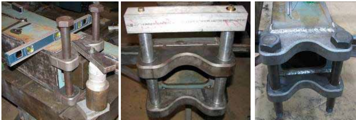
Figure 4.4: Left: clamping and jugging of Hinge Brackets. Middle: aluminum jig used to assure alignment. Welding was performed with jig in the holes. Right: finished Hinge Brackets with shoulder bolts in. The bolts should easily slide through holes when finished.
