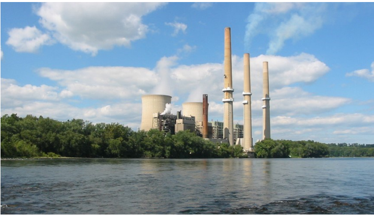
Martins Creek Power Plant, on the Delaware River, Bangor, Pa.
