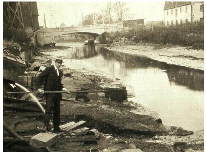
Bridgeport Canal up from Schuylkill River in 1928. (courtesy of the Phila. Water Dept.'s Historic Collection)
