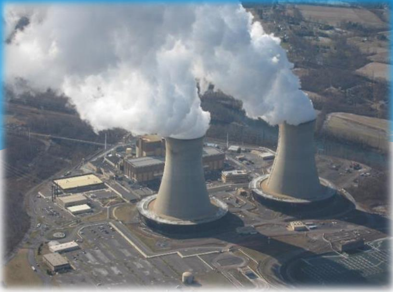
Exelon Limerick Generating Station, Montgomery County, Pa.
