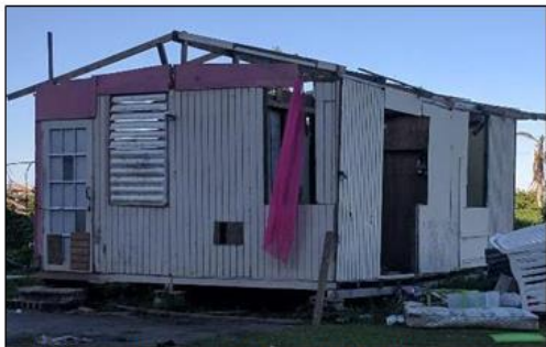
1 Story House: Wood Walls with Wood Roof
