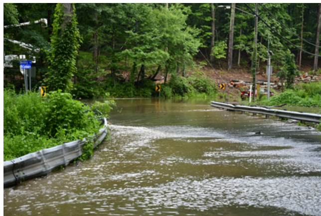
Heavy thunderstorms in Fairfax County, VA, on Aug. 5, 2022, added several inches of additional rainfall in less than three hours to already saturated ground, causing rapid rises in creeks and streams as well as flooding other low-lying areas.
