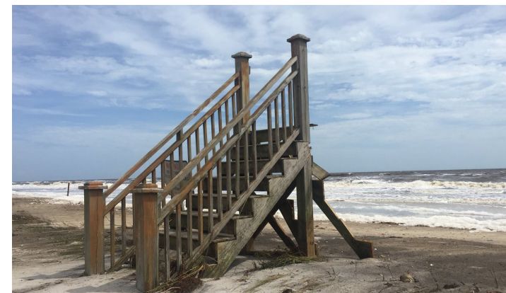
Wooden steps are all that's left of a pier in Newport, NC after Hurricane Florence made landfall in September 2018.
