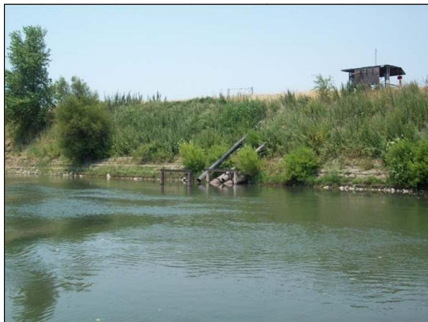
Figure 48. The South Steiner pump station intakes looking in a downstream direction.
