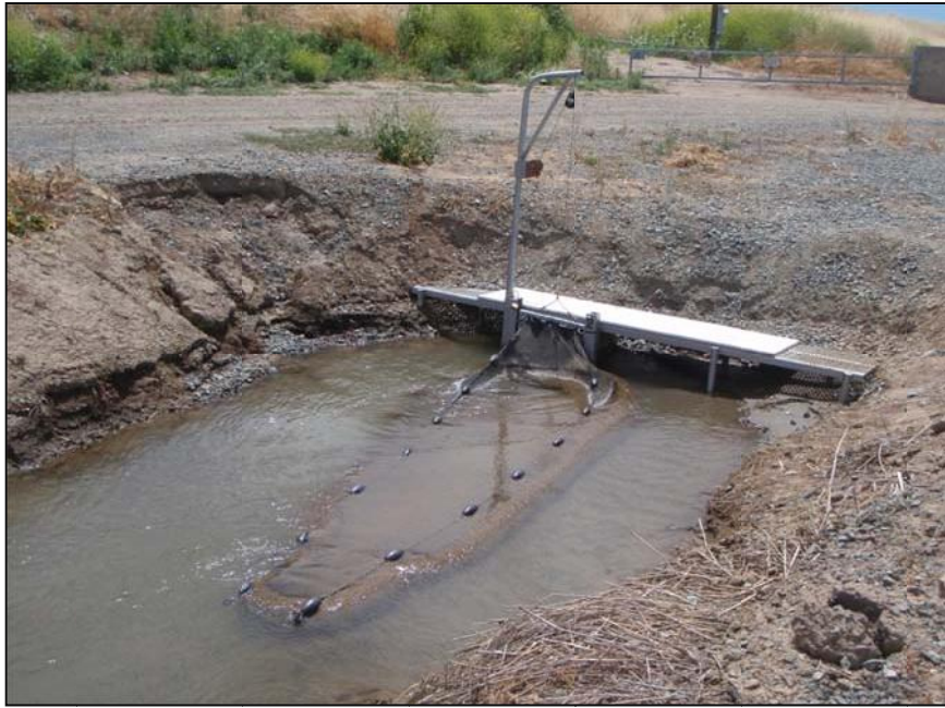
Figure 5. Fyke apparatus, fyke net, and sampling platform used to sample for fish entrainment in the South Steiner earth canal.
