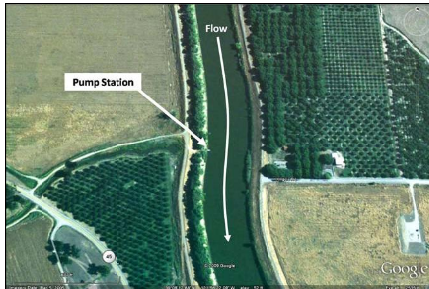
Figure 14. Location of the Sycamore pump station on the Sacramento River.
