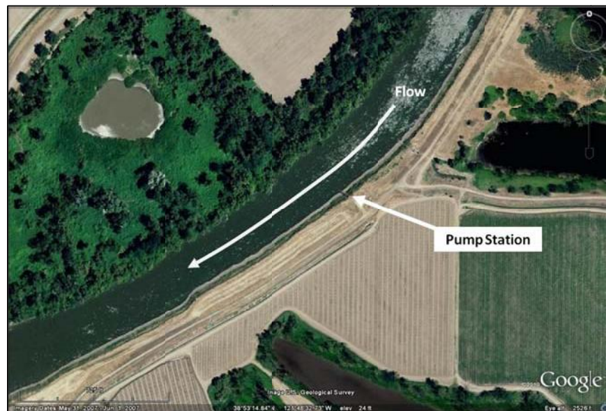
Figure 66. Location of the Windswept pump station on the Sacramento River.
