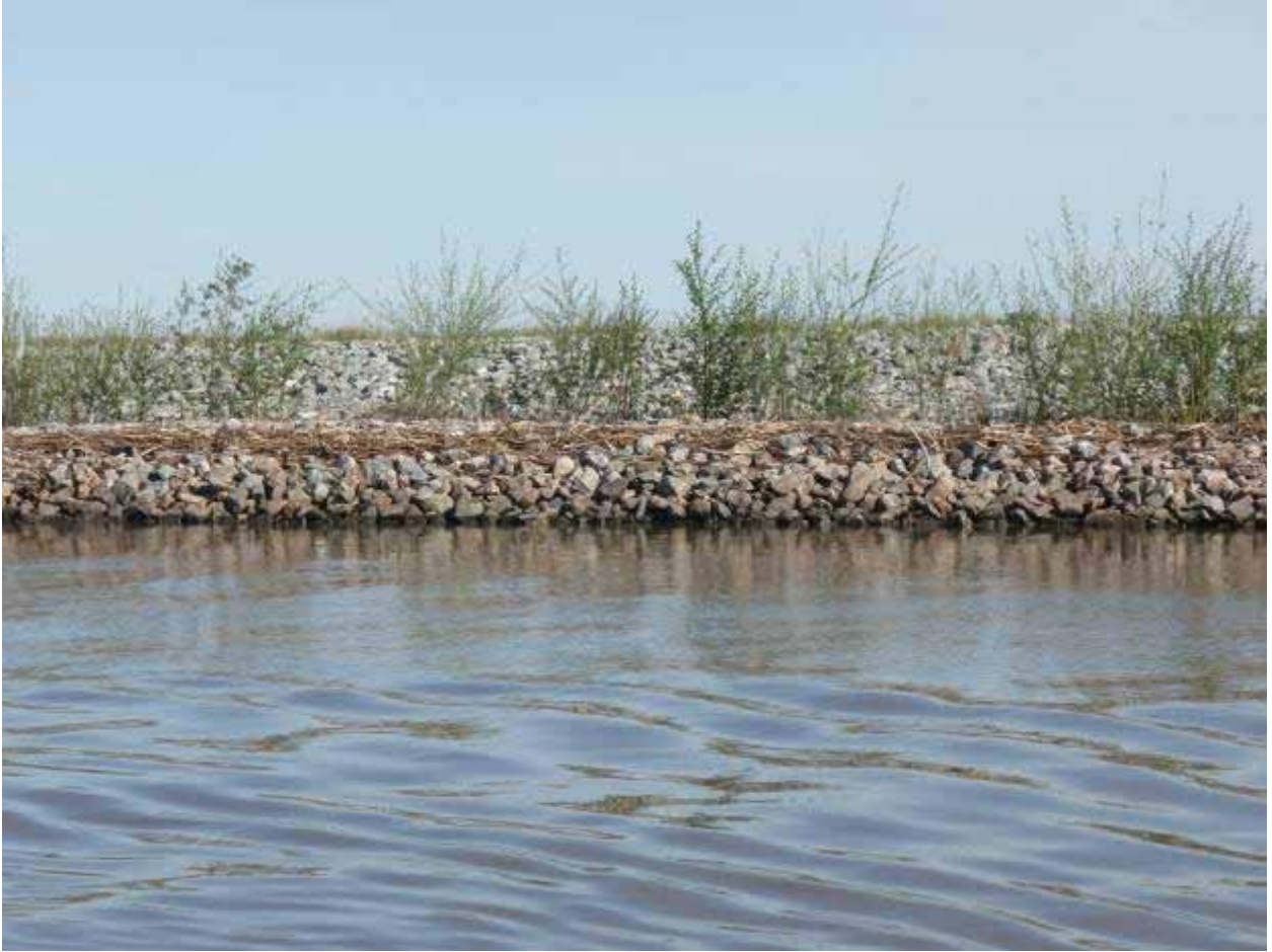
Figure C-7 - Upper Jones Tract, showing repair of 2004 breach with eco-bench
