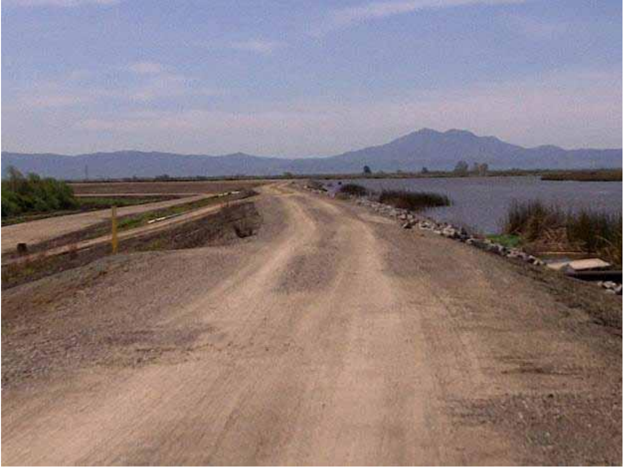
Figure C-9 - McDonald Island, showing PL 85-99 berm on landside
