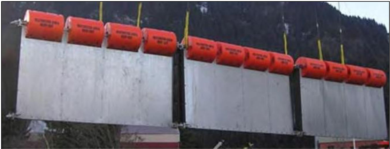
Figure 2-2 Three Sections of a Typical Floating Fish Guidance Structure
