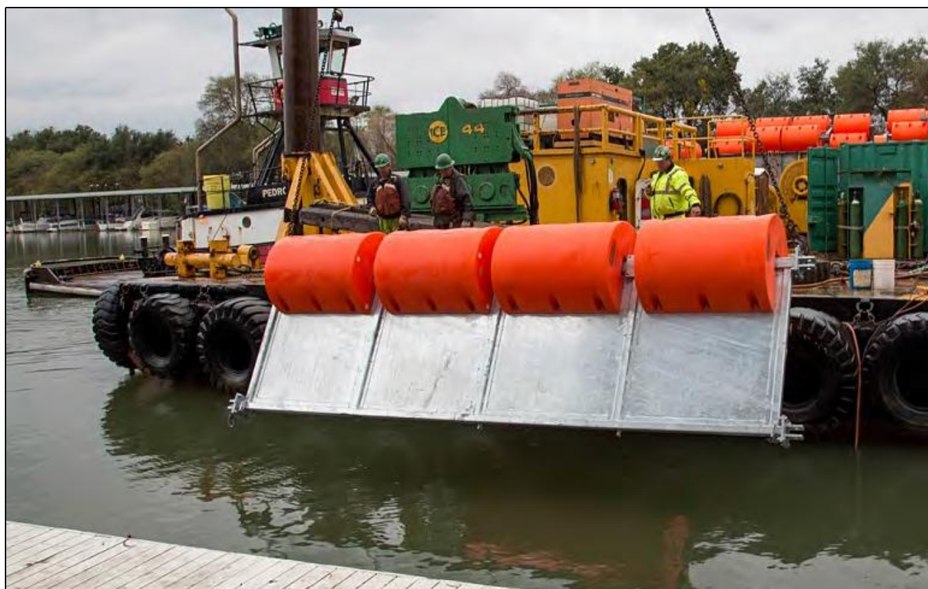
Figure 2-3 Georgiana Slough Floating Fish Guidance Structure Being Installed
