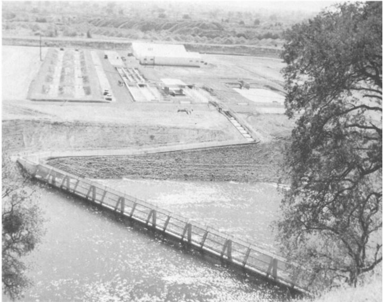
FIGURE 54. Nimbus Salmon and Steelhead Hatchery on the American River below Nimbus Dam, Sacramento County. Rack set diagonally across the river guides fish to the fish ladder entrance. Rearing ponds (empty when photograph was taken) at left. Hatchery and utility building at upper center. Adult holding ponds and spawning facilities at lower center. Mounds of gravel in the background are the result of gold dredging operations.
