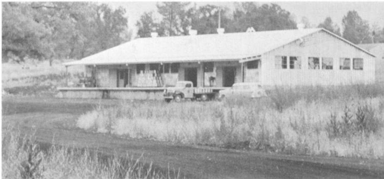
FIGURE 48. Feed storage and preparation room at Darrah Springs Hatchery. Constructed 1956, this building contains refrigeration and ice-making equipment.
