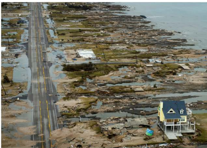
BOLIVAR PENINSULA IN TEXAS AFTER HURRICANE IKE (2008)
