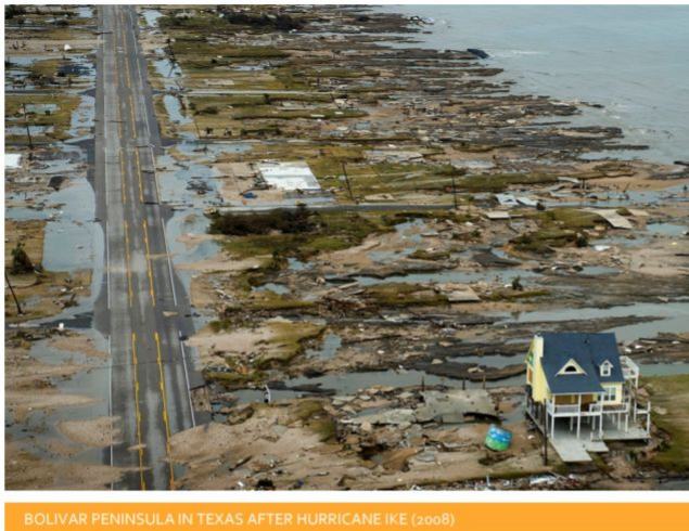
BOLIVAR PENINSULA IN TEXAS AFTER HURRICANE IKE (2008)
