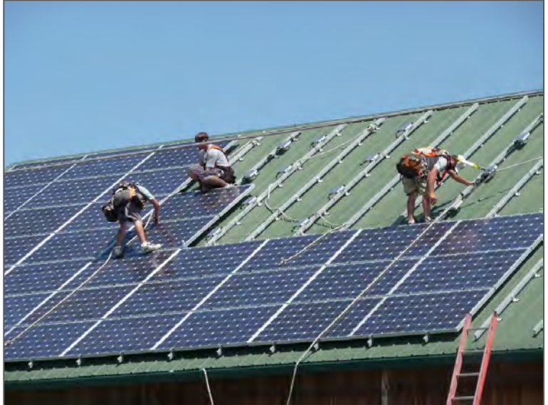
Installing solar panels on a barn roof →
